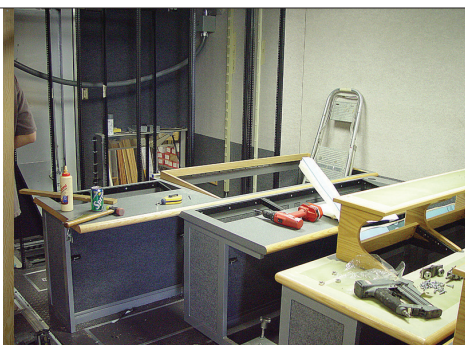
Figure 3.48 As walls and ceilings are completed, electrical distribution is being wrapped up.
